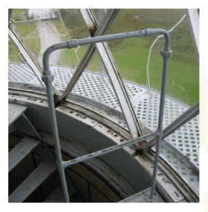
medium carbon steel is typically used for most AtoN applications today such as handrails, equipment brackets, new light support structures, etc.
